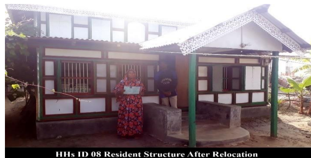
Photo 45: HH 08 after relocation in Polder-48
