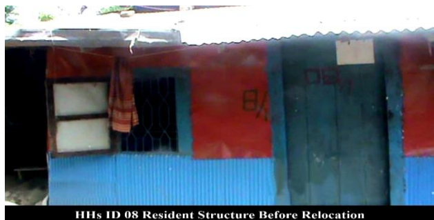
Photo 44: HH 08 before relocation in Polder-48
